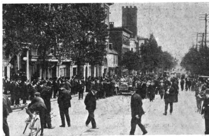
The Stop at the Official Control, Manalton House, Reading.
